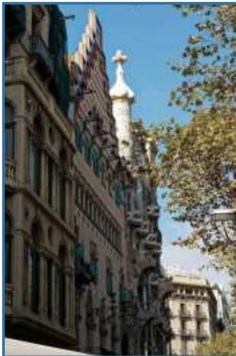
The undulating trencadís façade, with mask-balconies and the 'dragon' roof.
