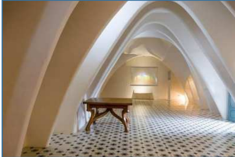
The attic of catenary arches, the 'skeleton' of the house of the dragon.
