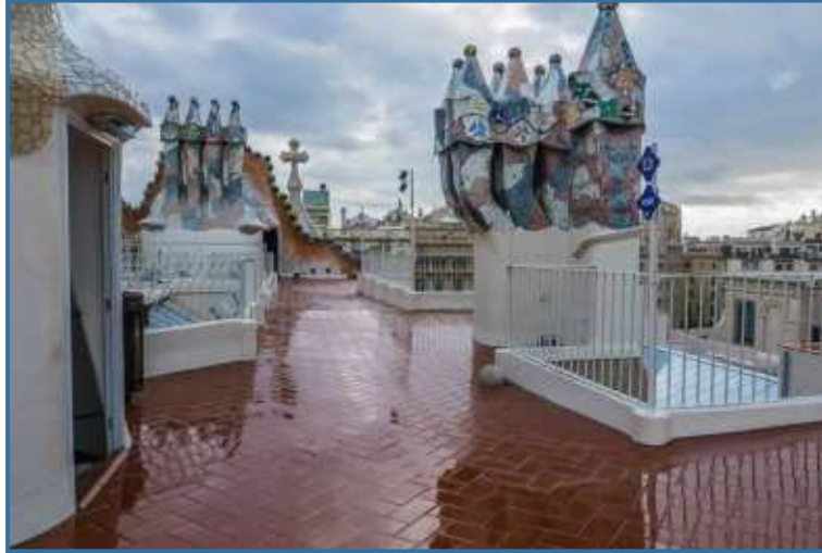
The trencadís chimneys and the scaly roof of the rooftop.
